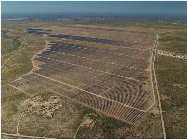
Located in Upton County in West Texas, the Roadrunner solar plus storage project is the largest operational solar project in Texas. (Photo: Enel Green Power)
